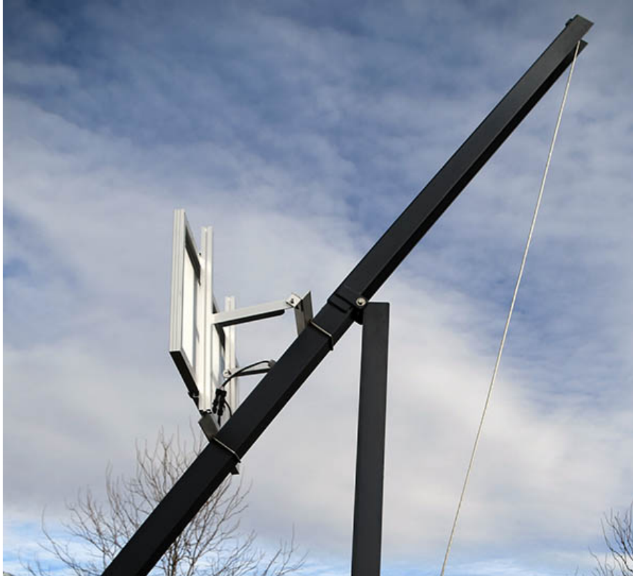
FIGURE 4-7 Solar Panel on Tip-Down Pole
