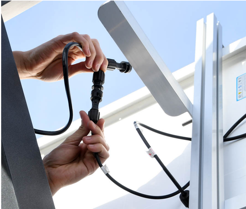
FIGURE 4-11 Connect Solar Cable to Panel
