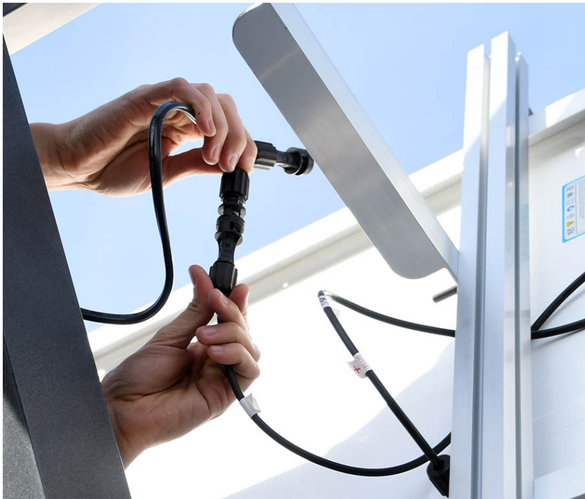
FIGURE 4-4 Connect Solar Cable to Panel
