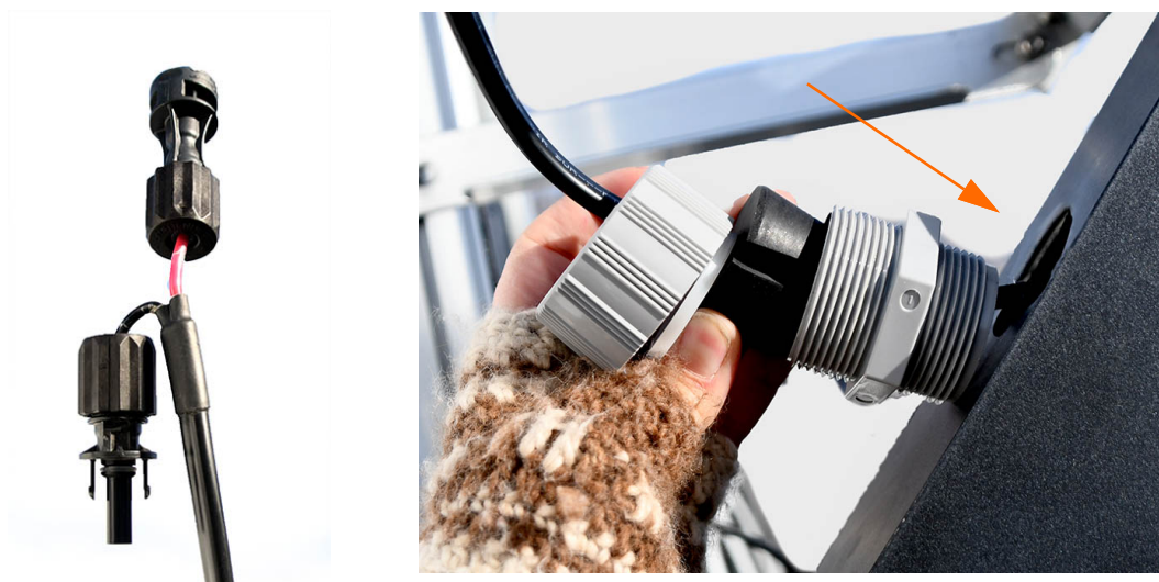
FIGURE 4-3 Gland Install
