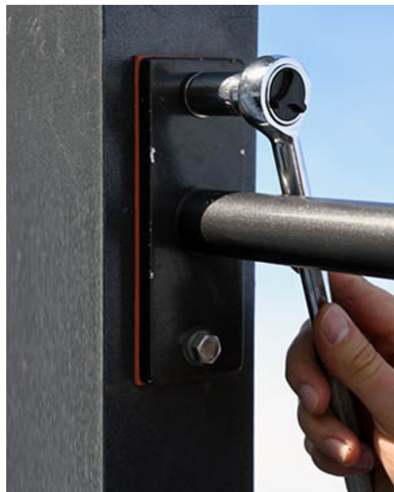
FIGURE 4-16 Weather Arm Bolted to the Pole
