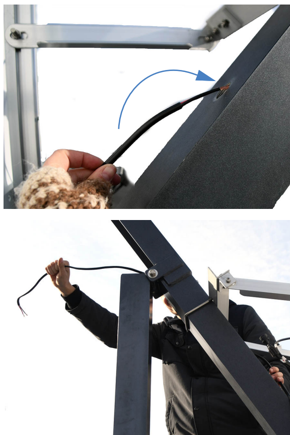
FIGURE 4-2 Feed Cable Down Pole
