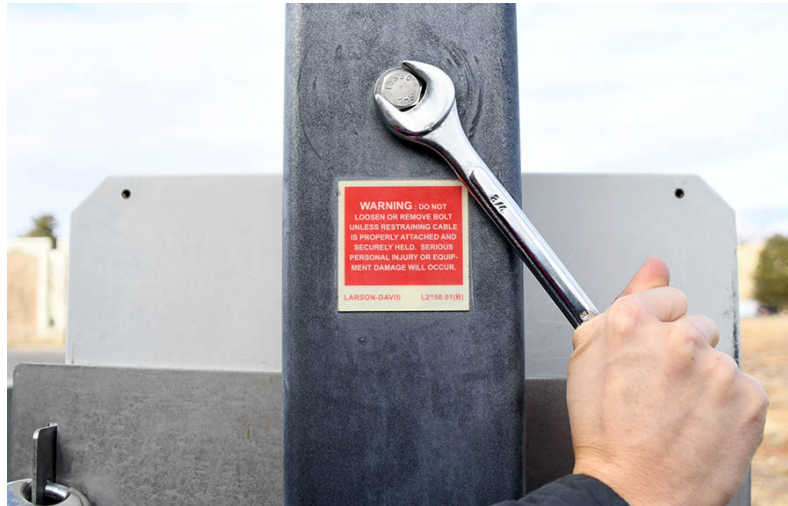
Figure 3-13 Removing Bolt from Pole
