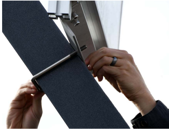
FIGURE 4-1 Solar Panel Install
